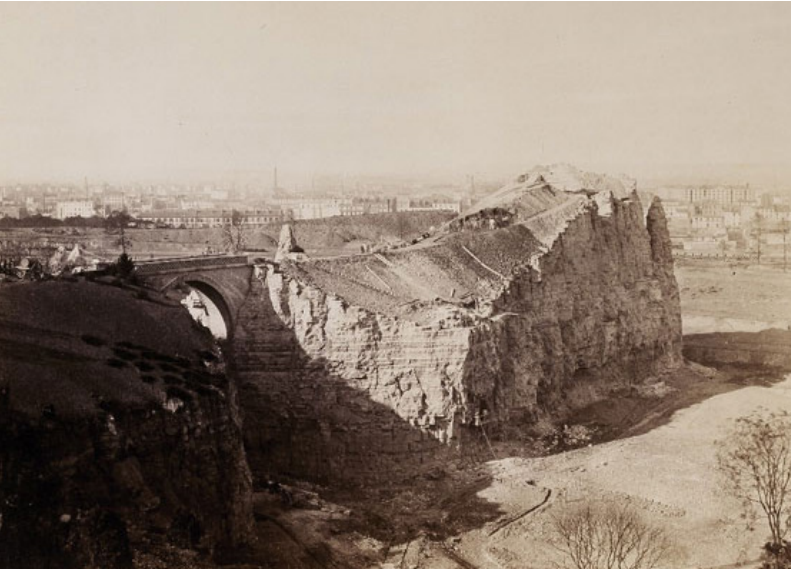
İnşaat halindeki park (1864–1867)
